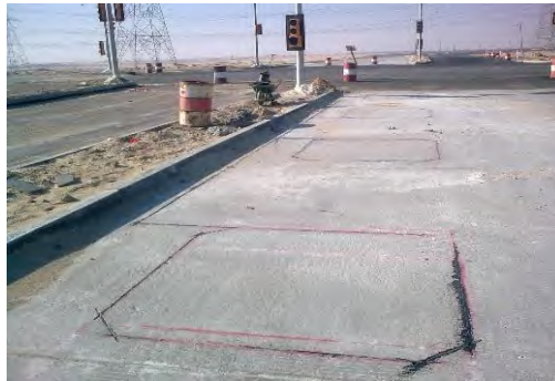
Traffic smart system detectors
