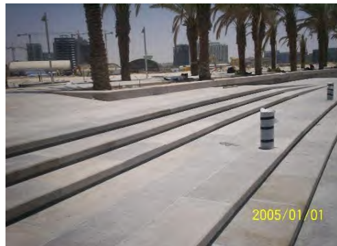
Ramps & Steps & Planters
