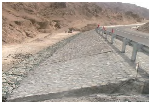
Slopes protection RIPRAP & Gabion
