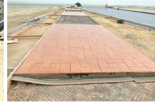
Walkways Stamped Concrete
