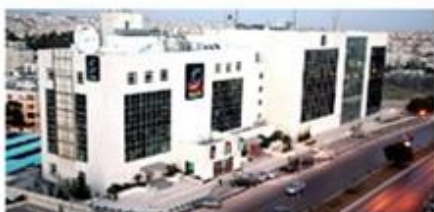
GSM Provider Power station
