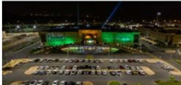
PSD -Telecom Servers Building
