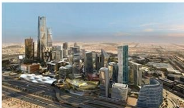
KAFD - Power Station Plant and infrastructure
