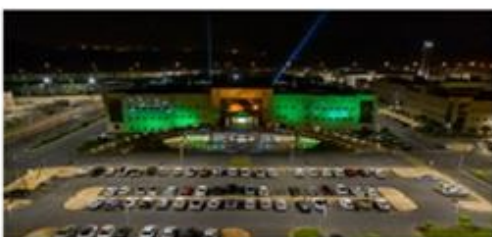
PSD -Telecom Servers Building
