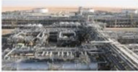
Khurais Gas Plant
