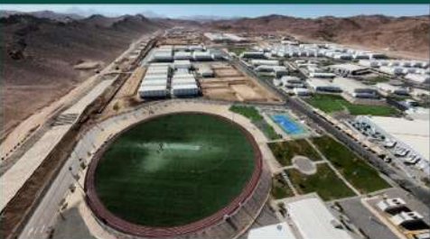
Neom Mountain Trojena Accommodations for Executive and Workers, Neom, Saudi Arabia
